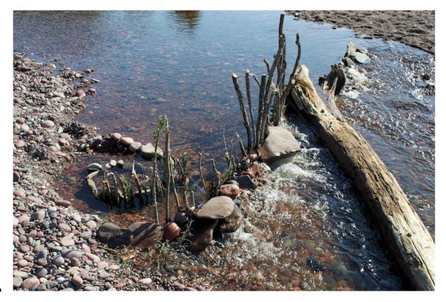
By blocking the entire width of the river, higher pressure risked washing away the spruce boughs. Bracing rocks against the back side prevented a potential washout.
