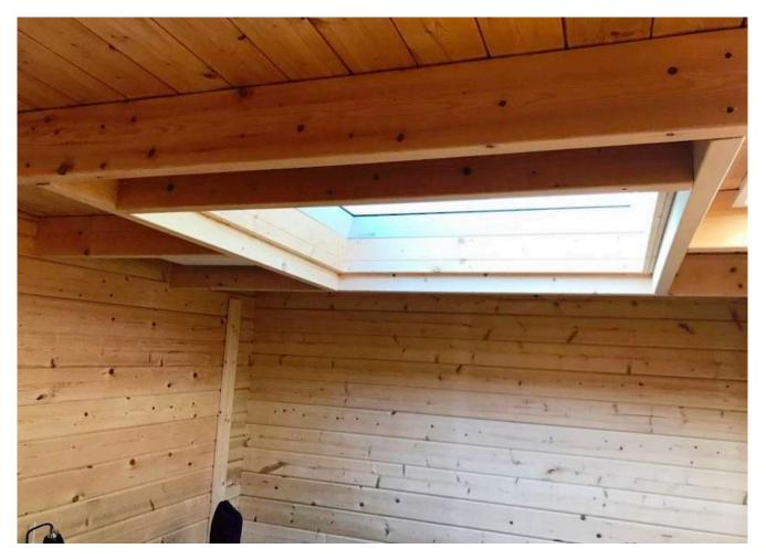
Drill a hole at the center of the location where you want to install the skylight, and then cut out the opening using a jigsaw or circular saw. Use some header joists to reinforce the rafters you just sawed off.
