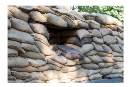
Hard cover is cover capable of stopping small arms fire such as steel-reinforced concrete, masonry, rock or two or more layers of sandbags. A certain amount of hard cover can be built ahead of time and then expanded up with sandbags as needed. Sand bags, of course, need sand, which can be stored in the form of a sand pit for kids to play in. Another solution is to remove sod and set it aside, dig a large hole, fill it with sand and then cover it over with top soil and replace the sod.
