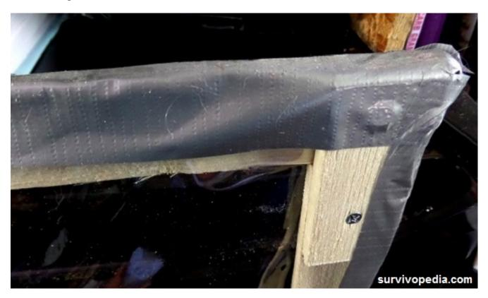
Step 2: Add additional layers of duct tape to fully secure vinyl to frame and also cut off any air pockets
