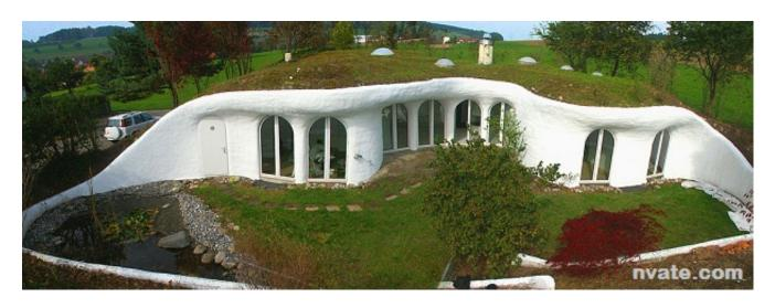
The home would stay cool in the summer, because of being underground and remain warmer in the winter, due to its ability to keep from losing heat. The ground around and over the home would act as excellent insulation to help the home maintain a comfortable temperature, year round.
